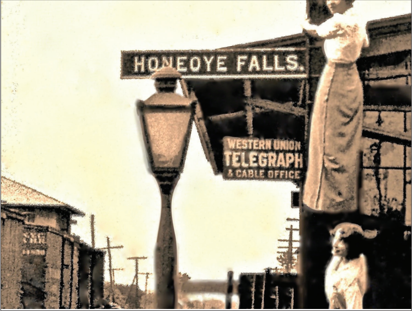
NYC depot sign was preserved... as a roof patch! (HF-Mendon Historical Society collection)
