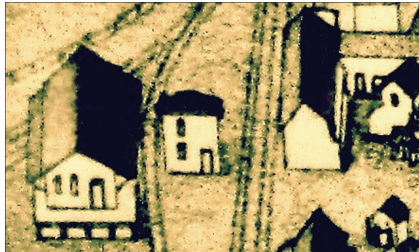
Bird's Eye zoom of the NYC's multi-functional freight house, pump station and west end of the Humphrey & Holdridge produce complex. The middle and eastern portion of the Humphrey building survives in 2023 - but barely. The freight house withered and was bullied to the ground thirty years ago. (Bird's Eye View, Burleigh Lithograph Co., Troy, NY 1892)
