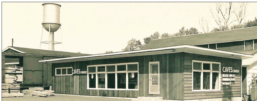
S. S. Caves Lumber , about the time of its store opening. To the left, note the railroad car, brimming with lumber, and the village water tower, another local 'Fallen Flag' in 1973.
